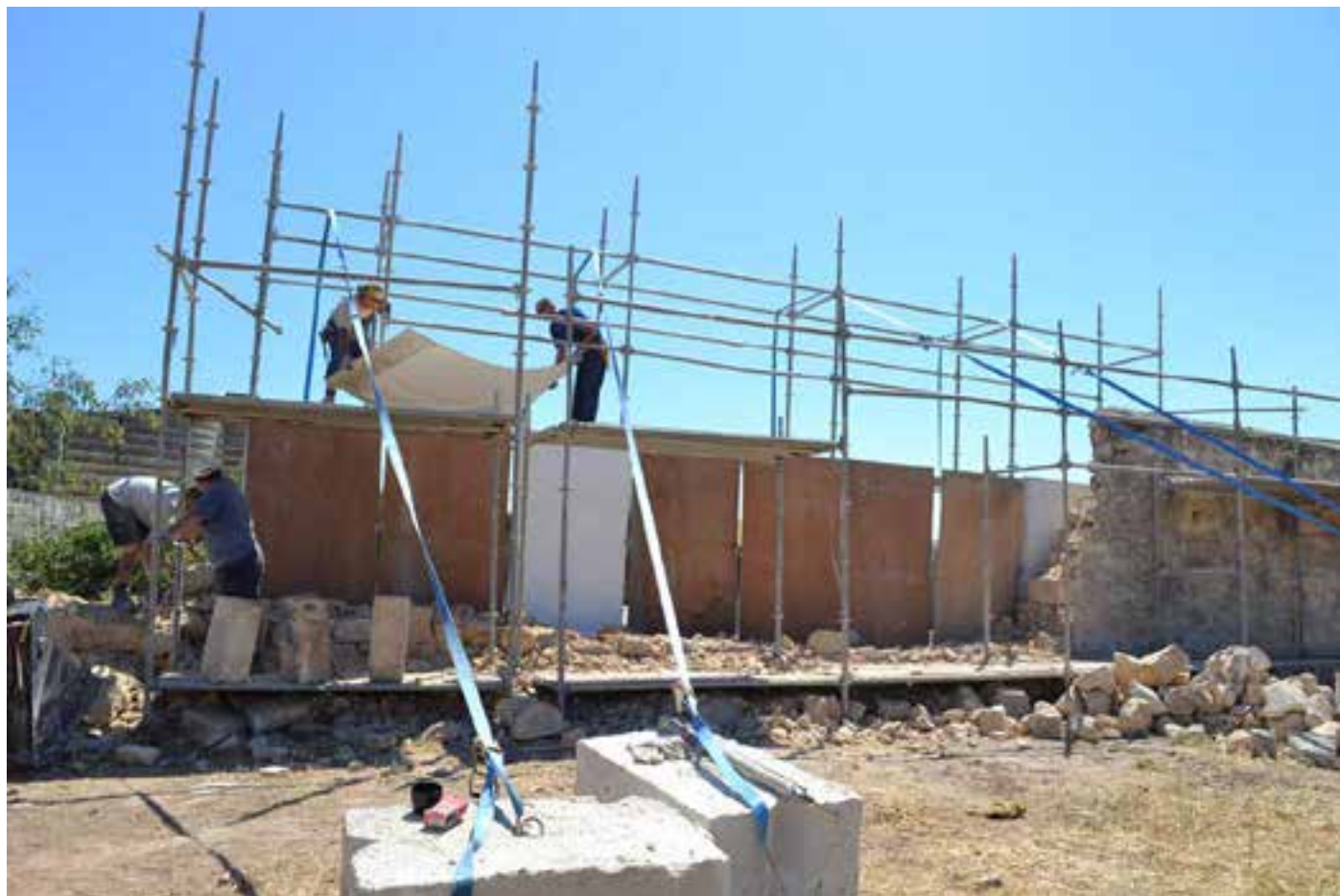
Demolishing of boundary wall between Temple site and back field with protective scaffolding installed to ensure safety of archaeological remains
